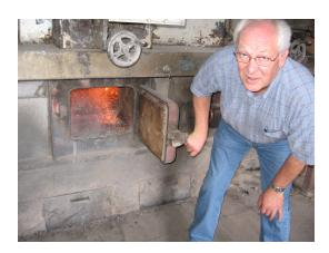
Aside from the labor needed for ash removal, the system is mostly automated and can be run practically unattended. Generally, about ten to fifteen hours per week are needed to operate the system.
